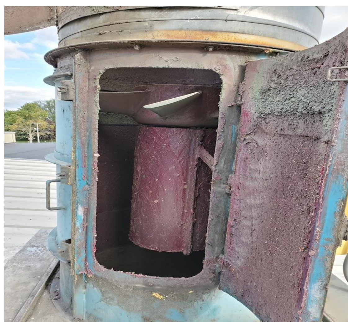
Figure 2: Paint Clogged Fan
